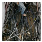
The wire phases are not color coded and need to be identified prior to termination
