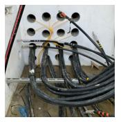
No factory installed SIMpull Head® pulling grips are installed at the end of the cable. The electrician will need to create pulling eyes using the strands of the cable
