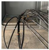
Each individual conductor was delivered on standard wooden reels. As a result, additional material handling was required.
