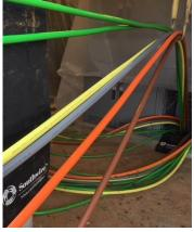
As cables entered the electrical room, they would encounter sharp corners that could potentially cause damage.
