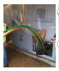
Cable needed to enter conduit without being damaged.
